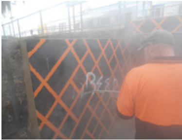
Removing graffiti off coated surfaces with pressure hot water
