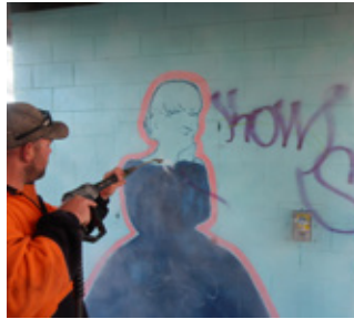
Removing graffiti off coated surfaces with pressure hot water
